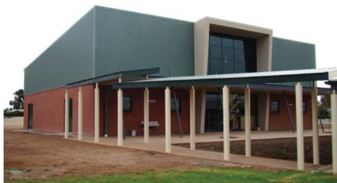
New assembly hall at Murray Bridge Christian College
