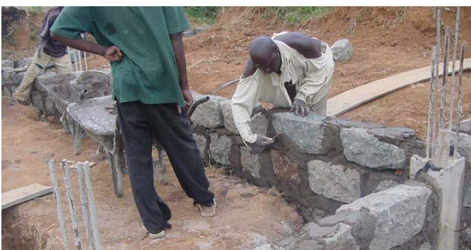
Construction work on Bethesda Girls High School
