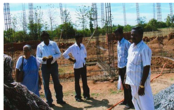
Building site for Christ Special School and Home
